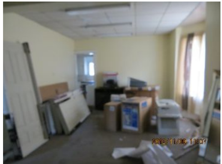
Interior Walls Condition
