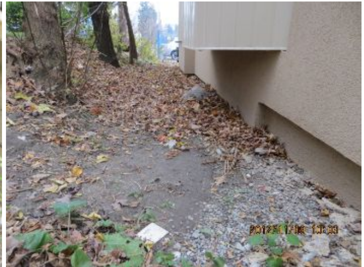
Sidewalk is pitched towards the structure, this may result in basement seepage. At east and rear
