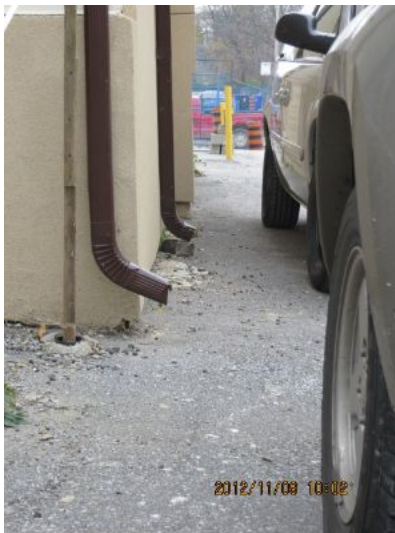
Extending all downspout(s) 4'-6' away from building.(All around the House)
