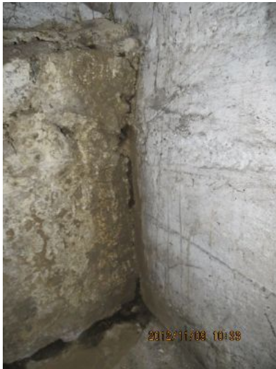
Active leaks observed at the time of inspection.
