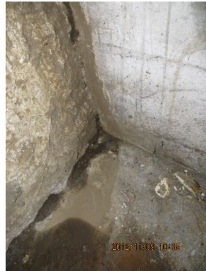
Active leaks observed at the time of inspection.
