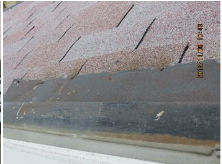
Flashing are original, recommend resealing/maintaining all flashings and through the roof vents as a part of routine maintenance. Recommended to be replaced in next roofing project.
