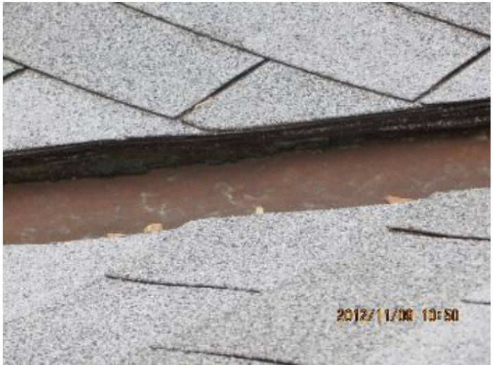
2 or more layers of shingles observed.
